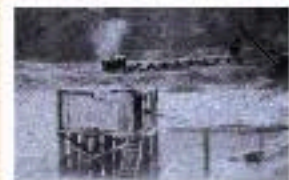
Excavating Waterfowl Lake was a grand effort. Train tracks were laid so that dirt could be transported away.
